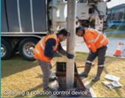
Cleaning a pollution control device.
